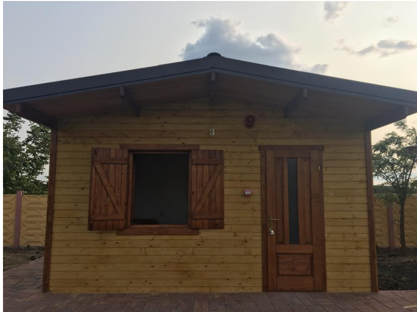
Figure 2. Accommodation Cabin Exterior
