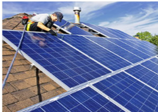
Figure 3. Photovoltaic Panel Installation
