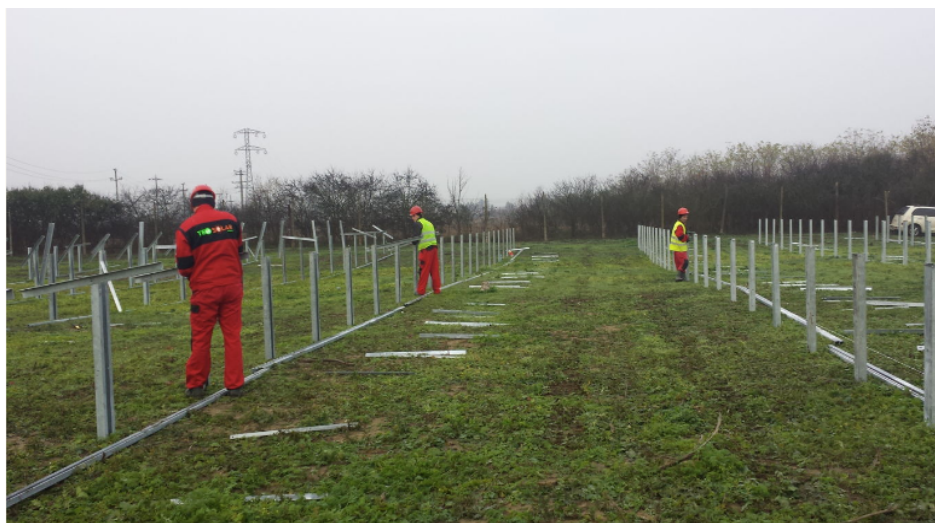
Figure 11. Installation of Panel Supports for a Photovoltaic Park in the City of Deta
