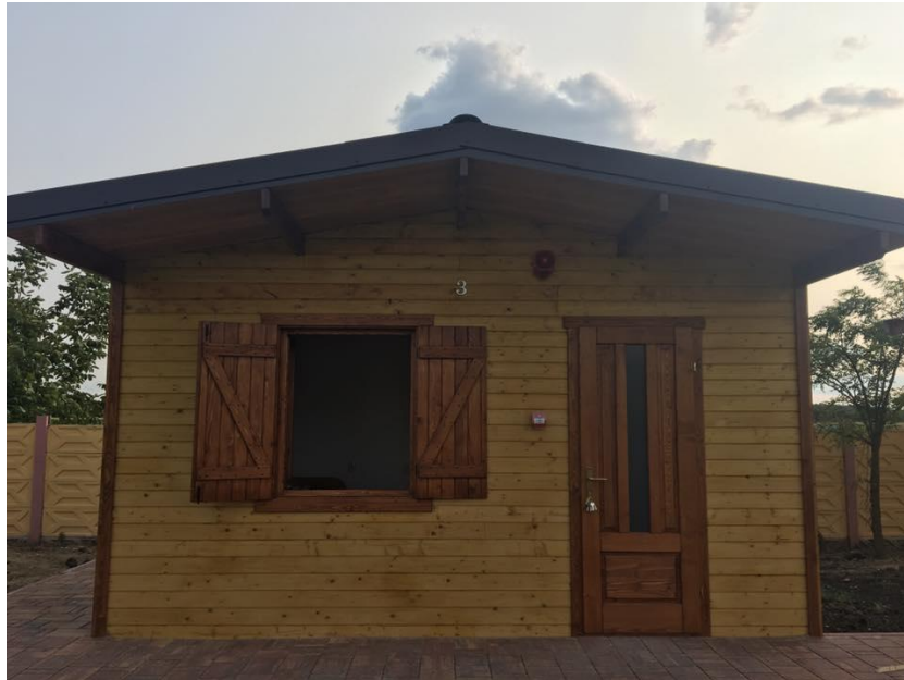
Figure 2. Accommodation Cabin Exterior
